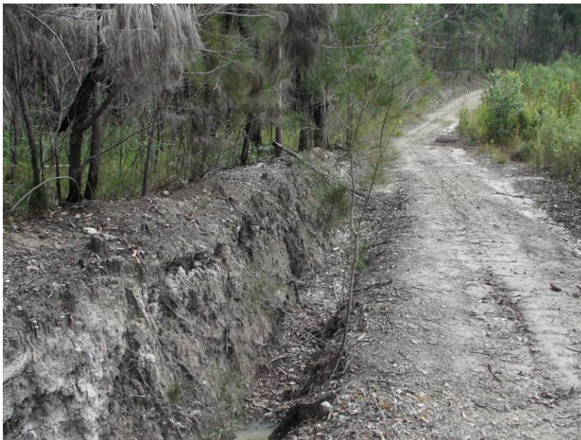
Plate 2: SU1 showing excavated drainage channels along existing dirt tracks – view to north.
